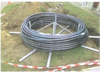
Fig. 2: A simple jig facilitates uncoiling of the flexible LPG piping on
